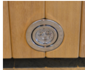
Side lighting - holes are cut into the side walls of the planter to allow LED spot lighting to be fitted.
