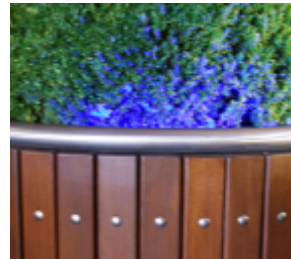
Up lighting - LED up lighting is fitted to the inside top of the planter, creating a rim of light between the planting and the planter
