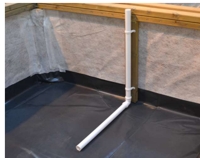
Polythene liner with filler pipe
