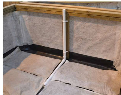
Hydroleca sacks laid out in base of planter
