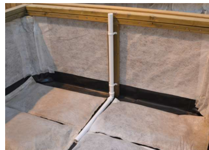
Hydroleca sacks laid out in base of planter
